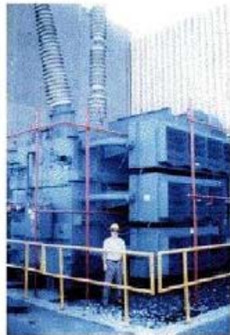
A large space storm in 1989 caused currents which damaged this transformer and shut off power for six million people for nine hours.
