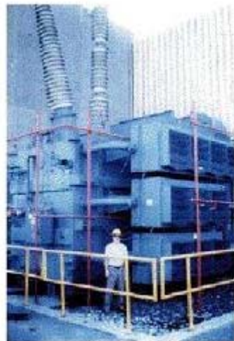
PJM Public Service Step Up Transformer Severe internal damage caused by the space storm of 13 March, 1989
